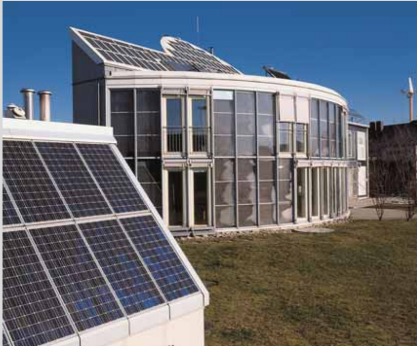
The Self-Sufficient Solar House Freiburg, DE 1992 Picture: triolog, Freiburg
